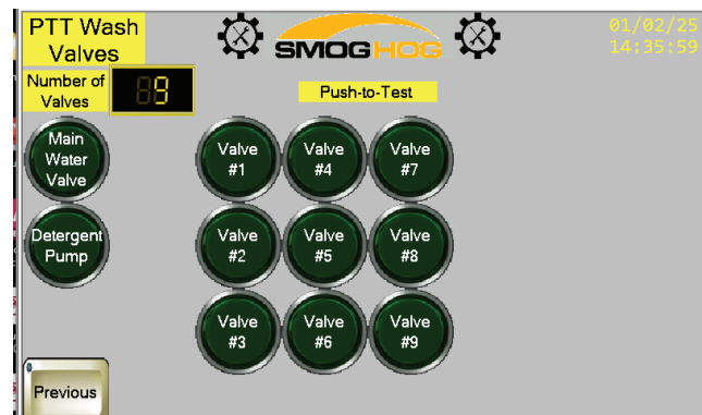
FIGURE 12. PTT Wash Valve Screen
