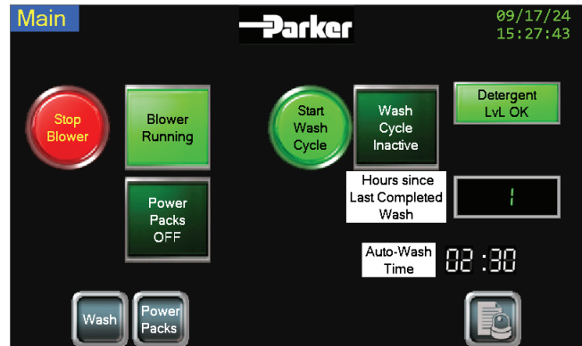
FIGURE 2. Main Operator Screen - Blower Running
